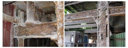
Fig. 3. View of the technical state of load-carrying beams and main beams of the frame
